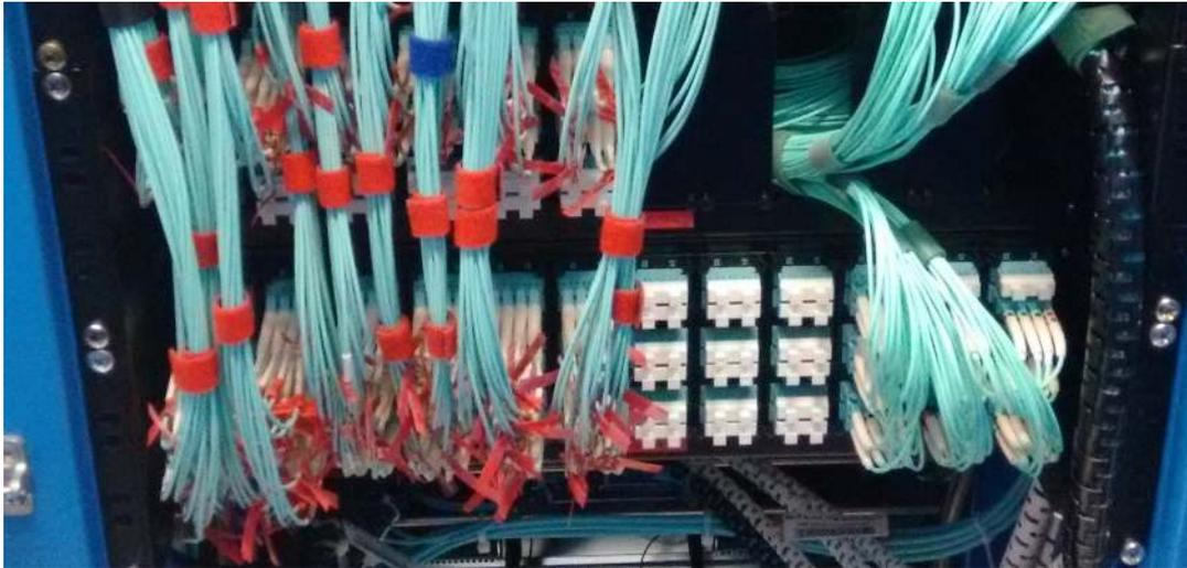
Figure B.1: Input BMTF fiber channels connected to the TwinMux patch panel
