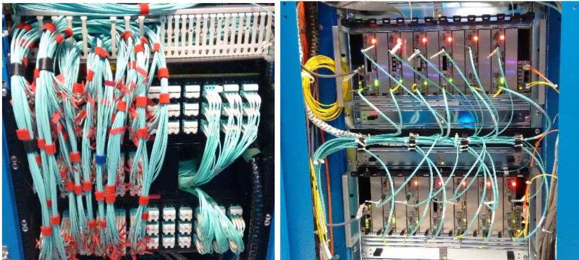
Figure 4.12: Left: 360 LC optical links are connected to the TwinMux patch panel carrying muon primitives to 12 BMTF processors (MP7 cards, right). Right: Each of the 12 trunk cables carries 30 LC links ( $12 \times 30 = 360$  overall) and is connected to the input of each of the 12 MP7s.
